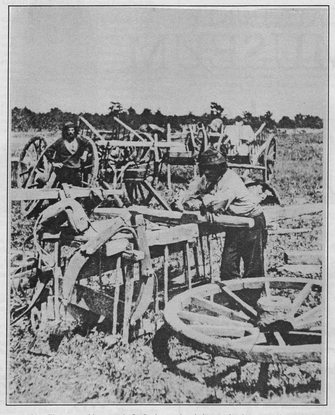
Repair time: These cart drivers are in St. Paul preparing their carts for the return trip north about 1858. The cart in the foreground has its wheels pulled off and is resting upside down. A new axle is in place. Note other spare axles laying around. A cart might go through four or five axles on a trip from Winnipeg to St. Paul.
