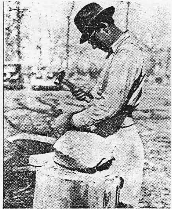
WPA worker Clifford Lenius of Dilworth uses a tree trunk bench, hammer and chisel to cut a field stone to shape, then tests his workmanship with a square. Fargo Forum photos by Roy Johnson.
